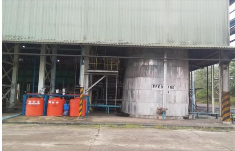
Gambar 1.2 Feed Tank Dari Area Water Treatment Plant
