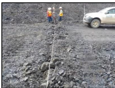
Gambar 2. Pengukuran Apparent Thickness
